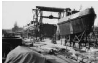
TID tugs have this hull shape because of the innovative method of their construction. The hulls were built in eight sections at inland engineering works. The sections were transported by lorry to the shipyards where they were welded together.
