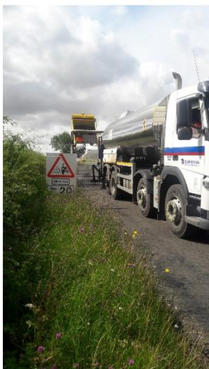
Treatments we might use range from full rebuilds (very expensive and only used where a road perhaps needs a reconstruction from its base), through machine resurfacing (not quite as expensive, but still not cheap – it's where we plane off the existing top layer and one or two new layers are added), through to techniques such as micro-surfacing and surface –dressing.
